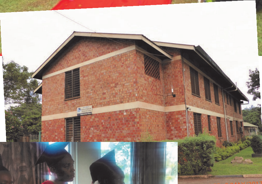
Rutwemba House—Education building
